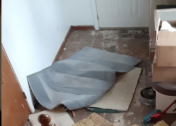
Sub-floor was totally rotted. Had to tear it up and replace it with \frac{3}{4} inch plywood
