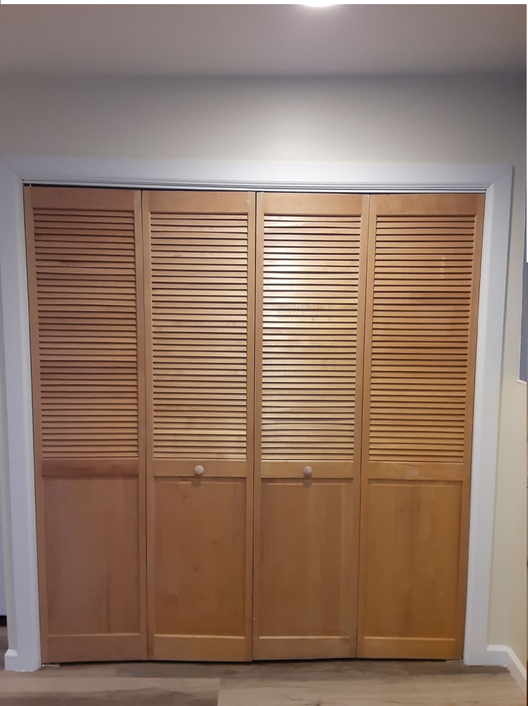
Built a closet and installed bi-fold doors
