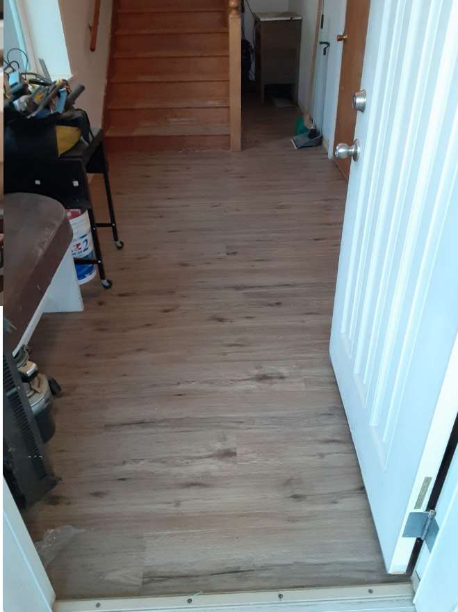
Installed new waterproof laminate/PVC flooring.
