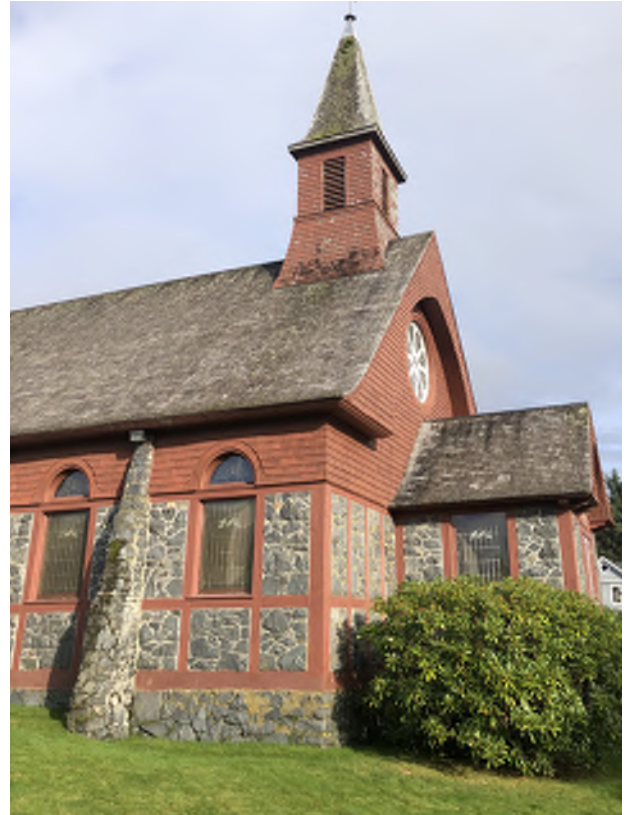
Figure 5.11: Timber lintels are continuous along the tops of the walls and divide the shingle siding and masonry.
