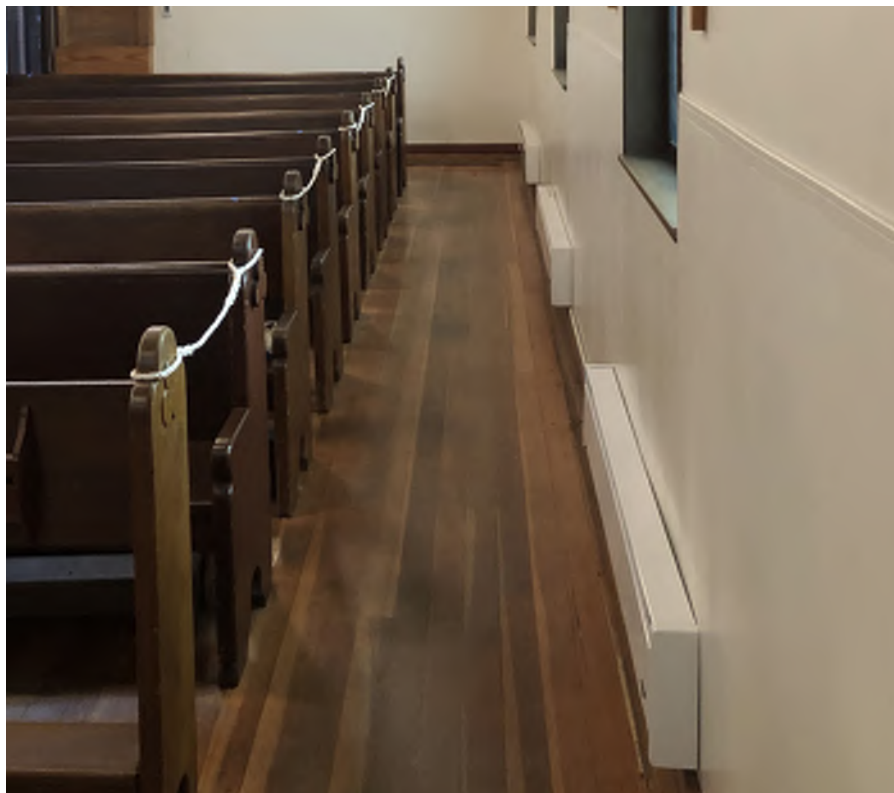
Figure 8.47: Baseboard heaters in sanctuary limit floor space.
