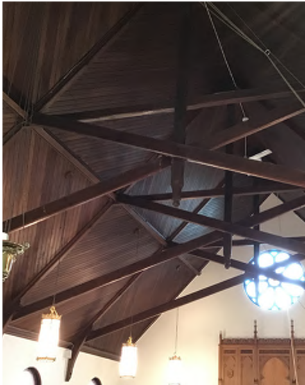
Figure 7.4: Exposed wood trusses, king posts with teardrop finials.
