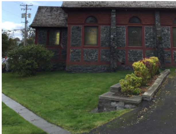
Figure 8.3: The drive also provides access to concrete pathways that connect parking to both the front and rear building entrances, looking southwest.
