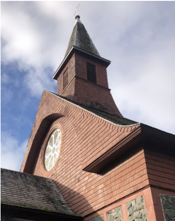
Figure 7.2: Steeply pitched roof with eaves, hooded arches at gable ends, belfry with pyramidal metal spires.
