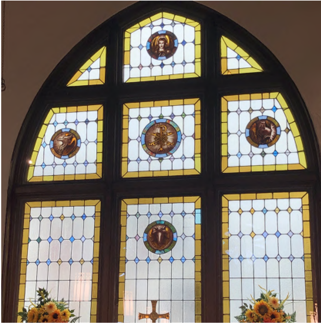
Figure 5.58: Detail of the north wall stained glass window assembly.
