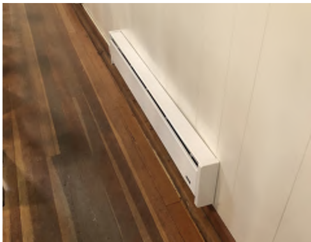
Figure 5.38: The wood floors at the east aisle. Also visible are the wall mounted heaters and the baseboards.
