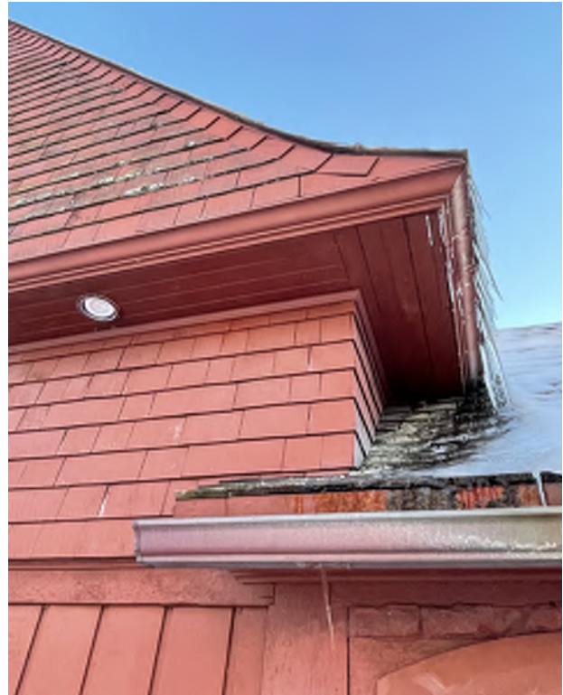
Figure 10.6: Install gutters on all roof sections. Photo credit: Troy Feller
