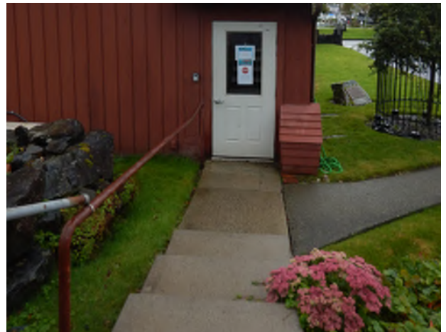
Figure 8.7: The concrete ramp/stairs have a metal pipe handrail on their east side.
