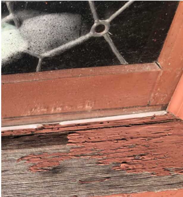
Figure 10.15: Remove clear sealant/caulking from the bottom of acrylic plastic coverings.
