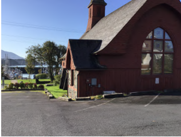
Figure 8.8: Designated van accessible parking space does not have an access aisle, and is not attached to a compliant accessible route connecting parking to building entry.
