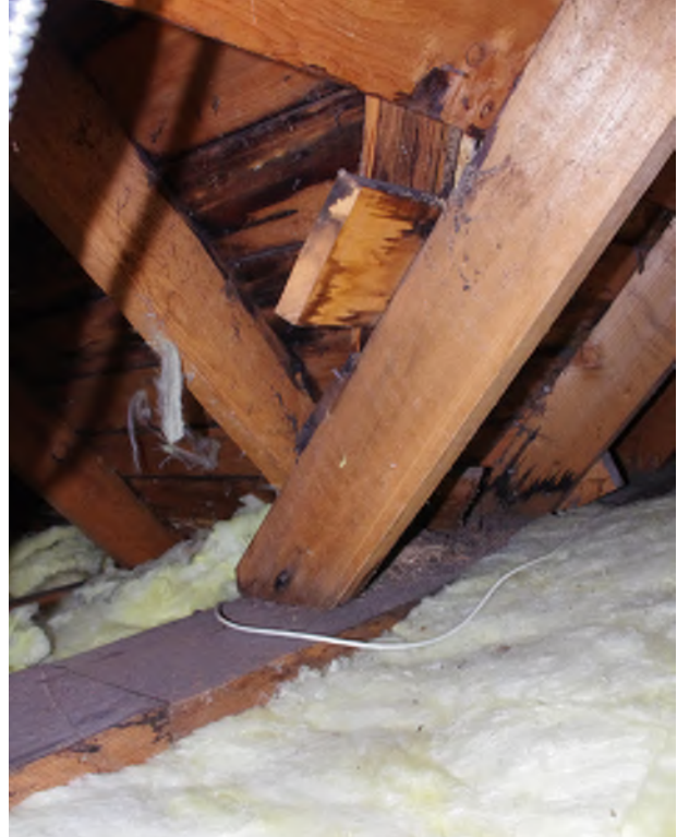
Figure 8.16: Roof rafter on top plate. Photo credit: Grant Crosby
