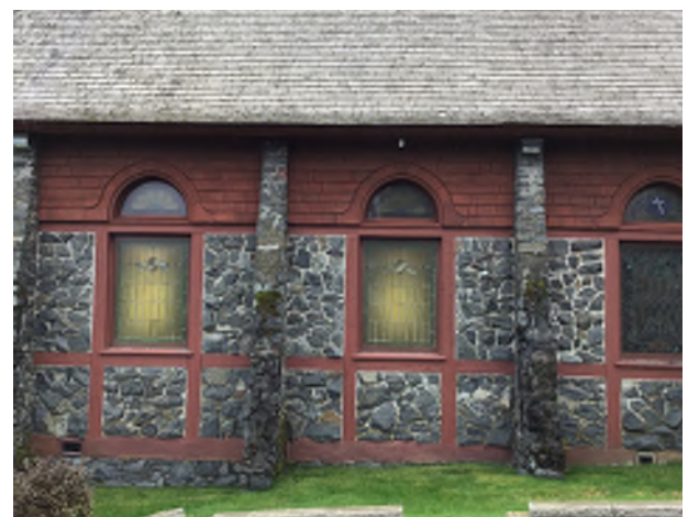
Figure 8.13: Typical half-timber framing positioned around windows centered in wall bays.
