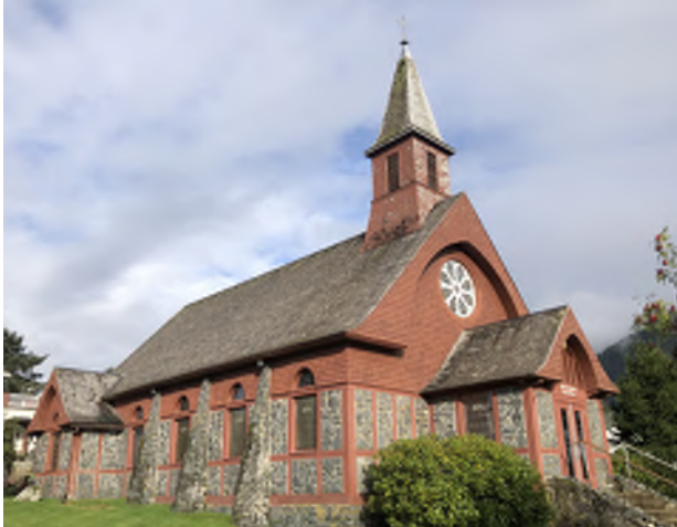
Figure 8.22: All roofs are sloped approximately 12:12 with flared eaves at lower ends.
