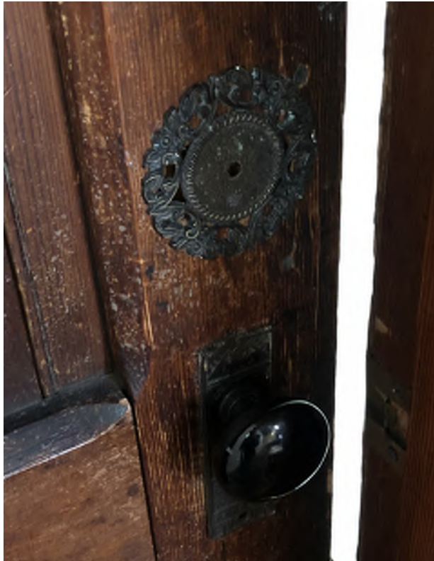
Figure 5.53: Detail of the original west transept door and hardware.
