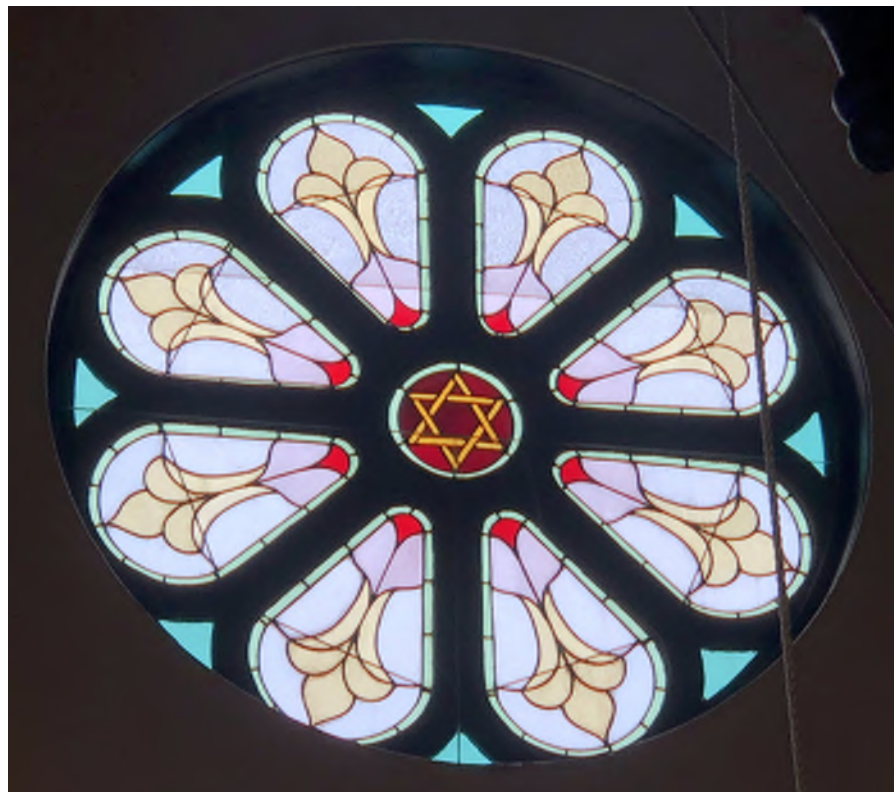
Figure 5.57: Detail of the rose window at the south gable of the church.
