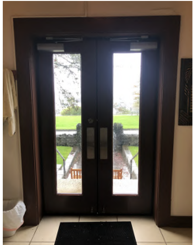
Figure 5.33: View of the church entry doors and the tile in the entry vestibule, looking south.
