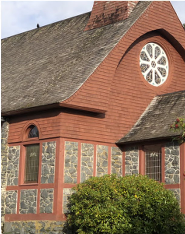
Figure 7.1: Half-timber framing and fieldstone wall infill at lower half of walls with painted wood shingles at upper half.
