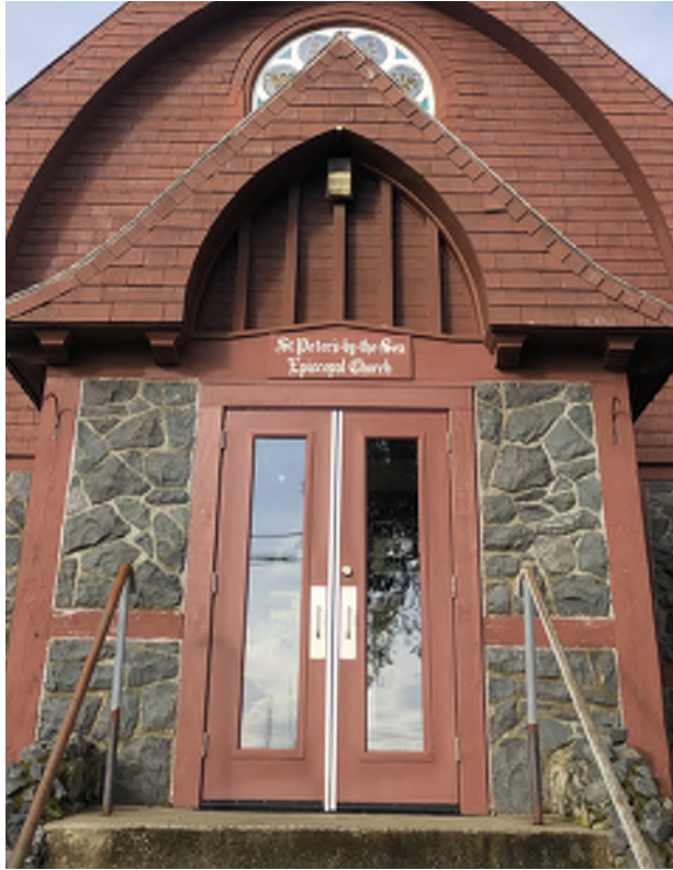
Figure 5.24: Entrance doors are glazed metal-skinned doors that are not original.
