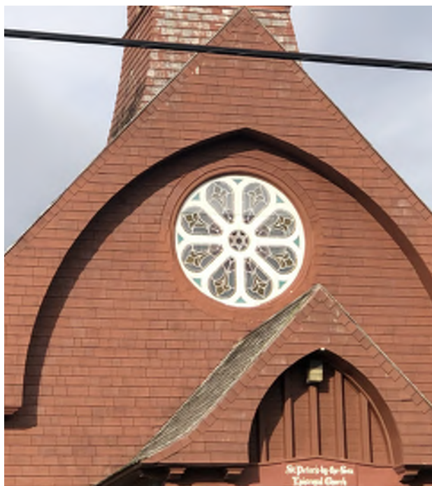
Figure 5.20: The large rose window at the south front facade features eight, teardrop shaped lites filled with floral patterns.
