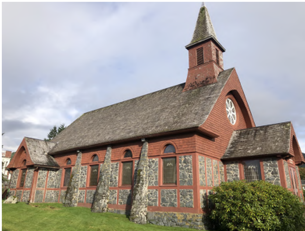
Figure 5.12: The church has a steeply pitched, gable roof with the ridge oriented perpendicular to Lincoln Street, and lower cross gables over transepts run parallel to the street, looking northeast.
