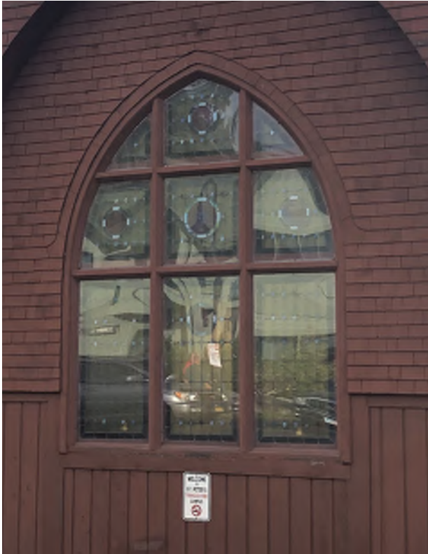
Figure 5.29: A large, nine-panel stained-glass, pointed arch window dominates the north facade.
