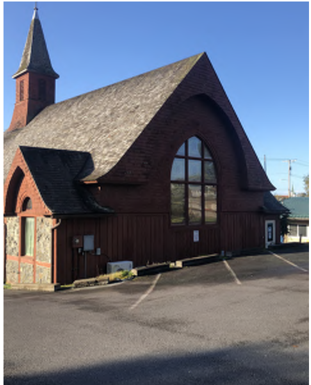
Figure 5.5: Paved parking to the north of the church, looking southwest.
