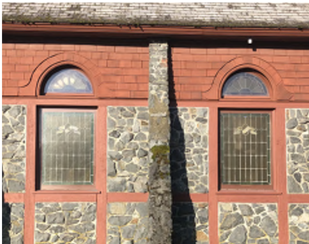
Figure 8.40: Typical windows of lower sash rectangular leaded stained glass windows with an upper semicircular leaded glass transom on the east and west facades.
