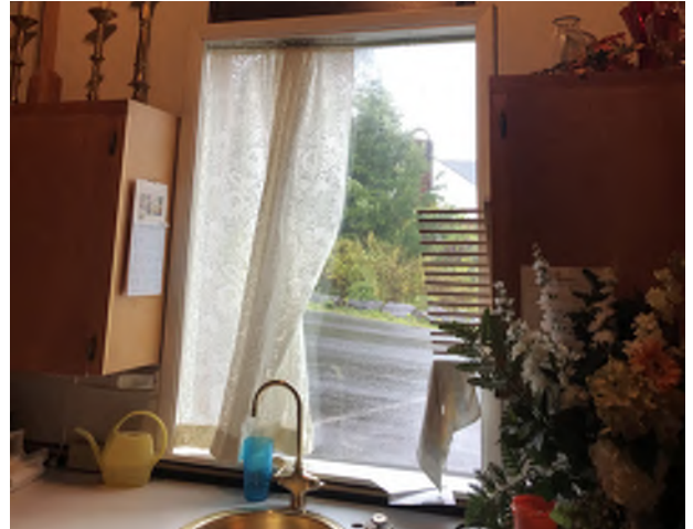
Figure 5.50: Detail of the altered window in the east transept, looking east.
