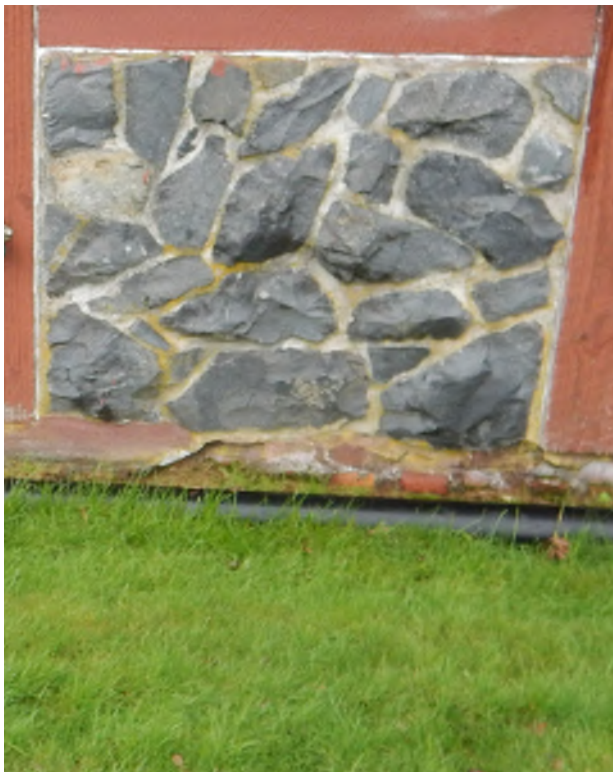
Figure 10.5: Patch and repair mortar parge coat on brick foundation walls.
