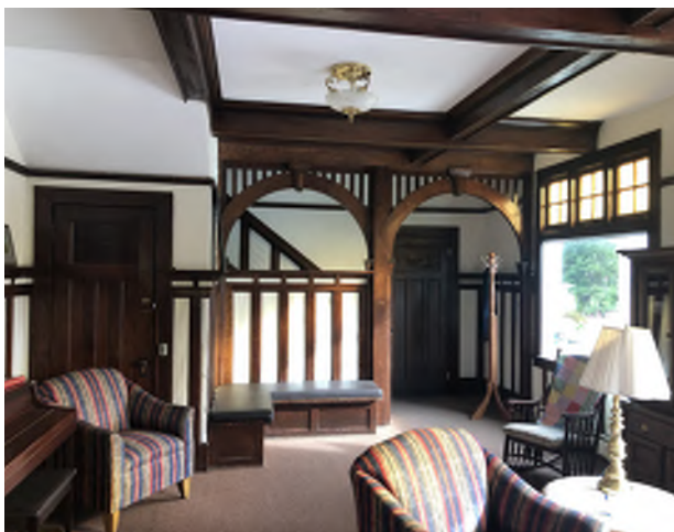
Figure 8.34: Intact plaster wall finish with original wood wainscoting in Living Room.
