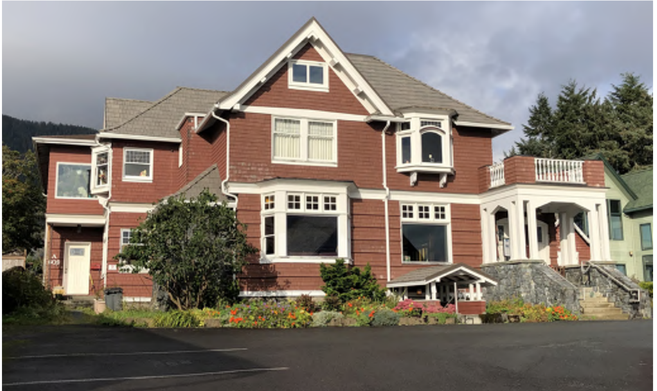
Figure 5.10: Overview of See House, looking north.
