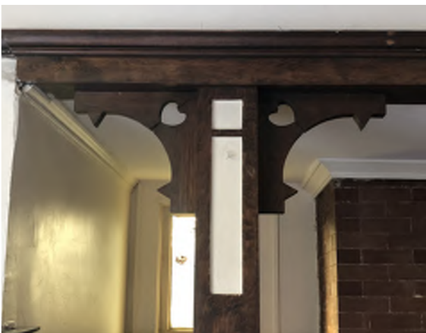
Figure 5.44: Inglenook columns with decorative heart-shaped cut outs.
