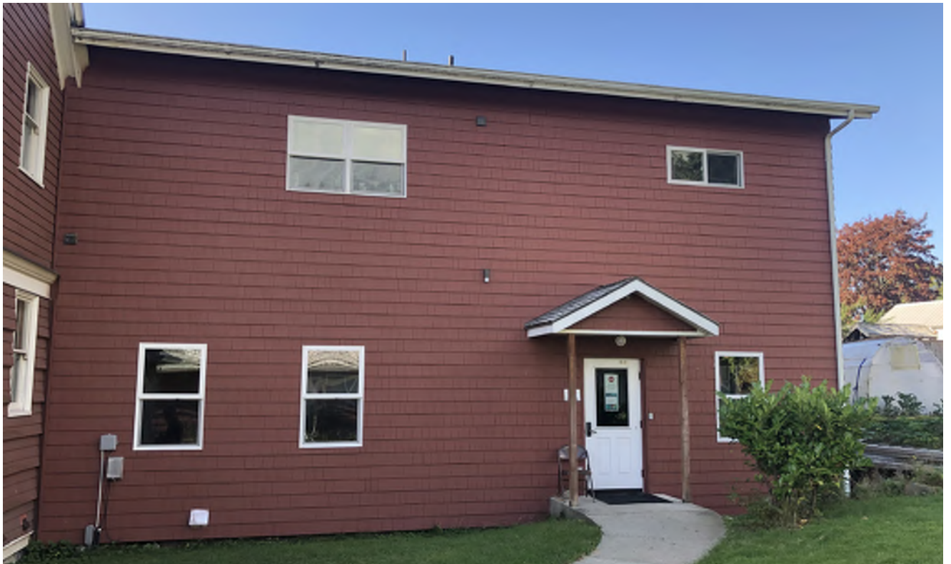
Figure 5.32: The east façade of the 1956 addition, looking west.
