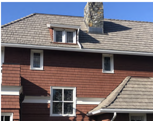
Figure 5.27: The central section of the east façade with the four-lite stained glass window, dormer and chimney.
