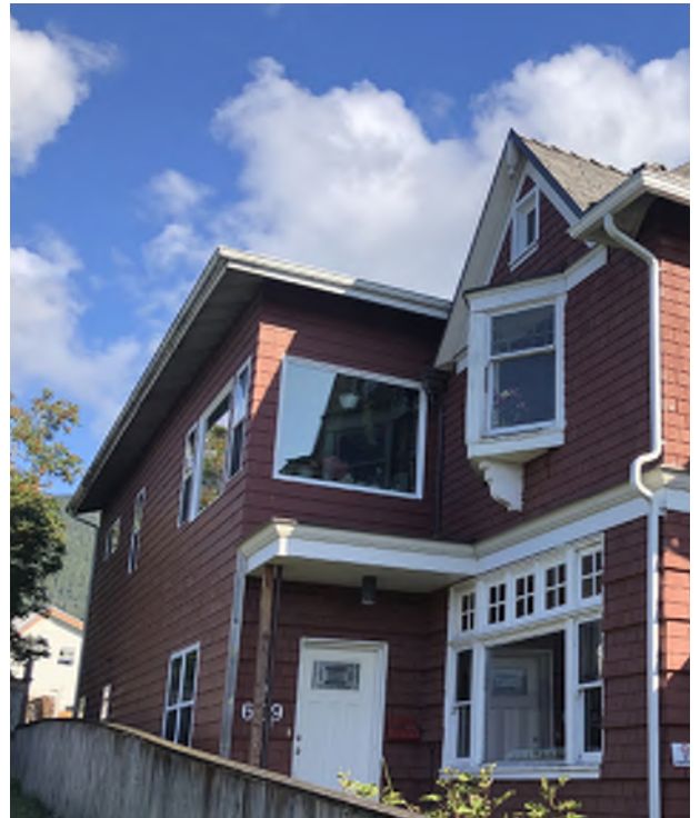
Figure 5.33: West façade of the 1956 addition, looking northeast.
