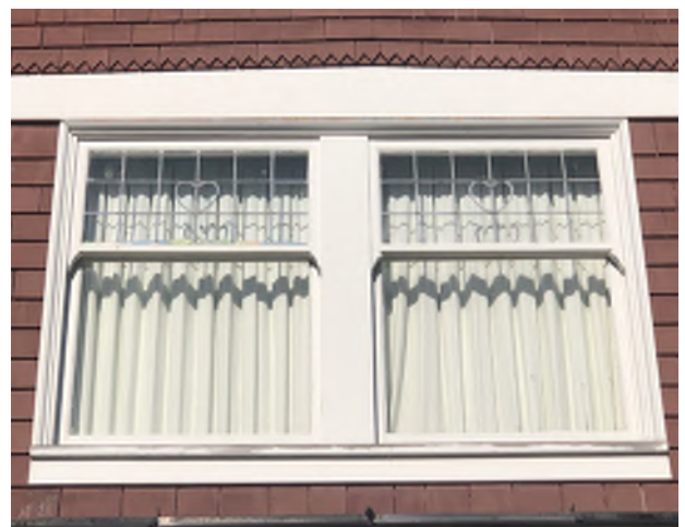
Figure 5.18: Detail of the typical leaded windows with the heart motif.
