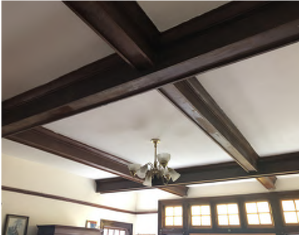
Figure 5.42: Plaster ceilings with dark-stained wood beams in the Living Room.
