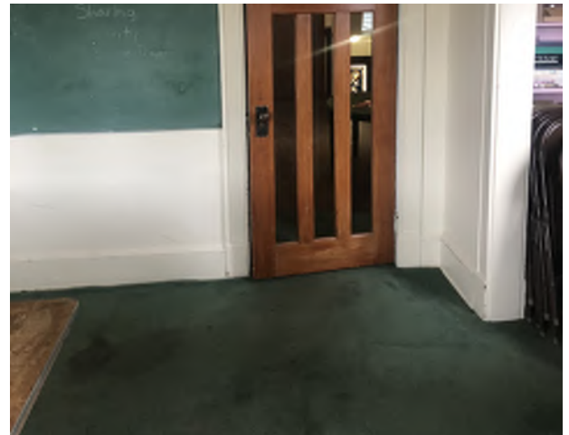
Figure 5.63: The door and carpet in the northwest bedroom (Bishop's Bedroom).
