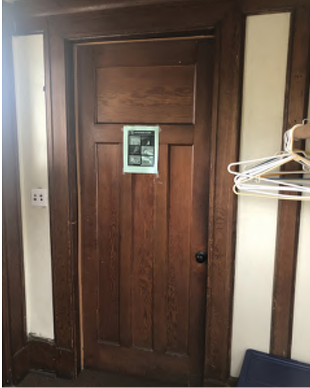
Figure 8.45: Original Vestibule door that leads to the Living Room.
