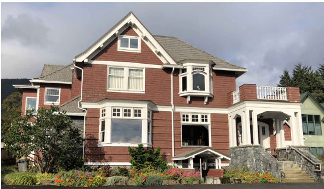
Figure 8.9: Synthetic (plastic) shakes have replaced the original cedar shingle roof.
