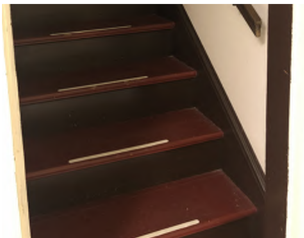
Figure 5.53: Secondary stair to second story hallway, accessed from the Kitchen.
