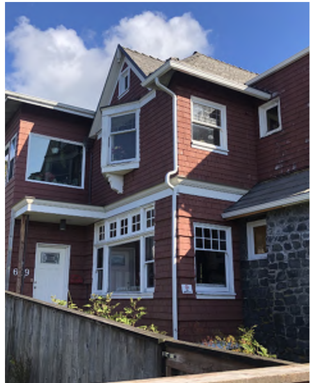
Figure 5.24: Overview of the west façade, looking northeast.
