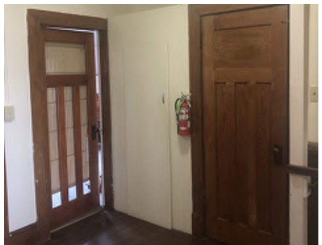
Figure 5.56: The Attic, closet and northeast corner bedroom doorways off the hallway.
