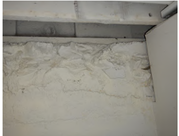
Figure 8.6: The concrete stem wall foundation topped with 1 to 3 feet of rubble masonry.
