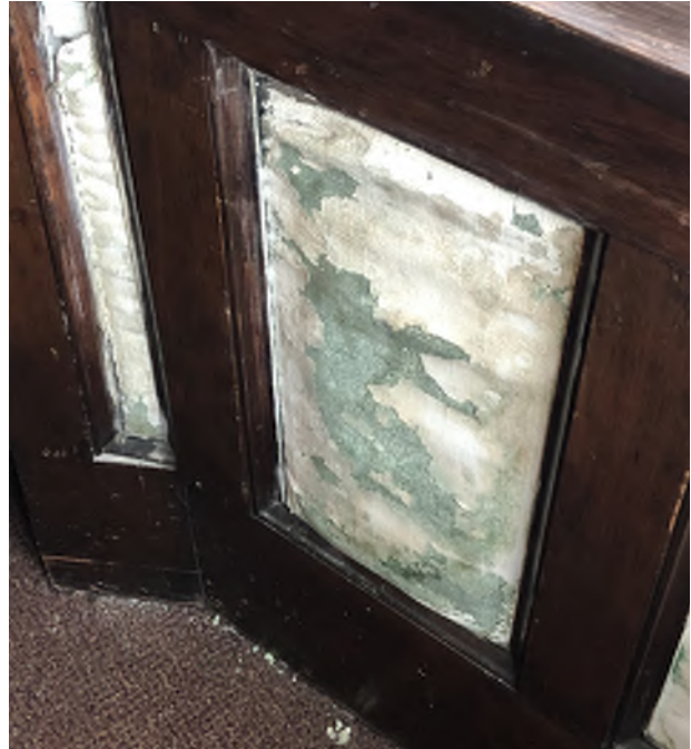
Figure 10.20: Restore damaged plaster and/or burlap wall finishes.
