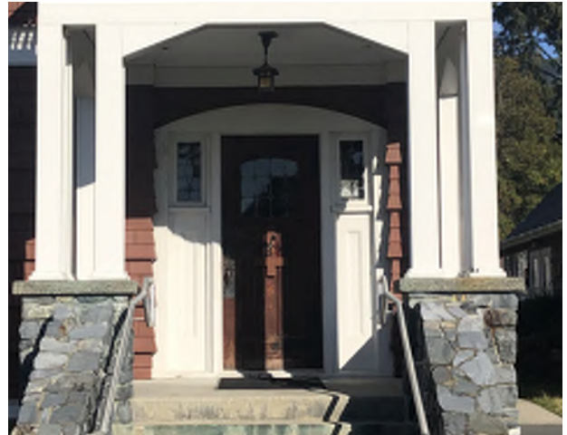
Figure 8.23: Primary entrance and entrance door accessed through covered porch and concrete stairs.
