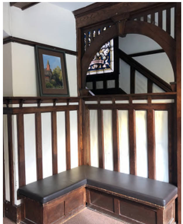
Figure 5.39: Wood arched entryway with keystone motif and simple wood slats.
