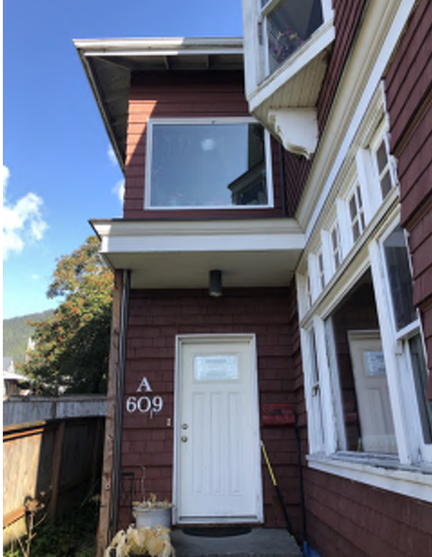
Figure 5.31: South facade of the 1956 Fellowship Hall addition, which provides the entry to the apartment, looking north.
