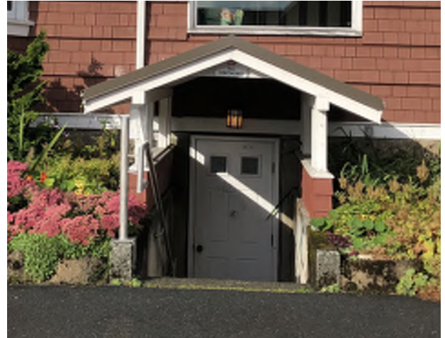
Figure 5.16: The addition of the fixed awning at the basement level entry, looking north.
