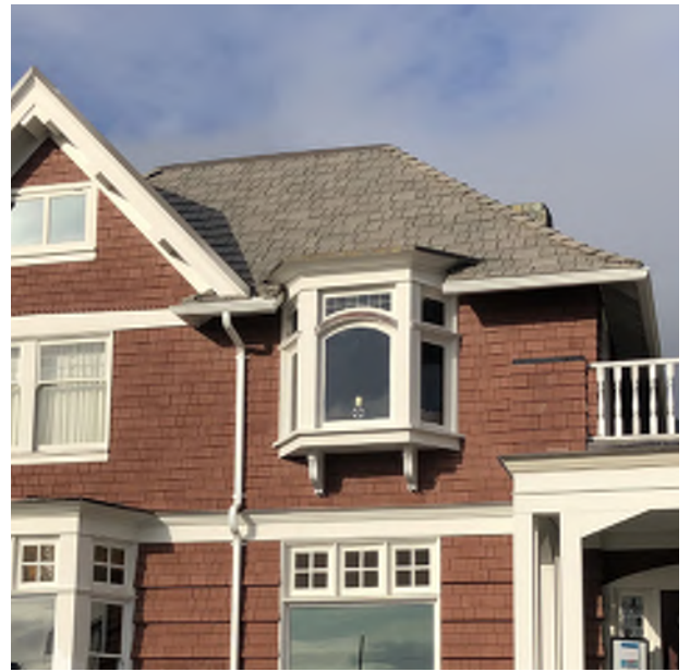
Figure 9.2: Materials are largely intact or replaced in kind, with exception of the synthetic roofing shingles.
