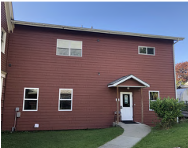
Figure 5.8: Pathway between the rear addition of the See House and the Archives Building, looking west.
