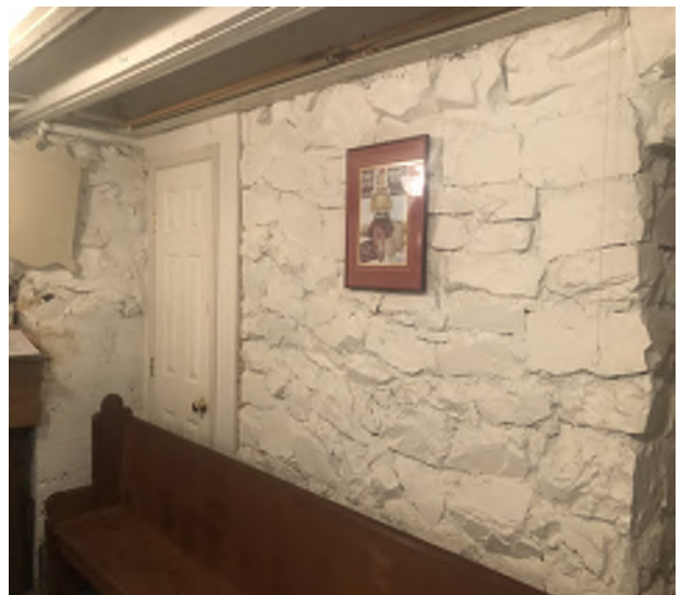
Figure 5.76: The painted stone wall at the Basement.
