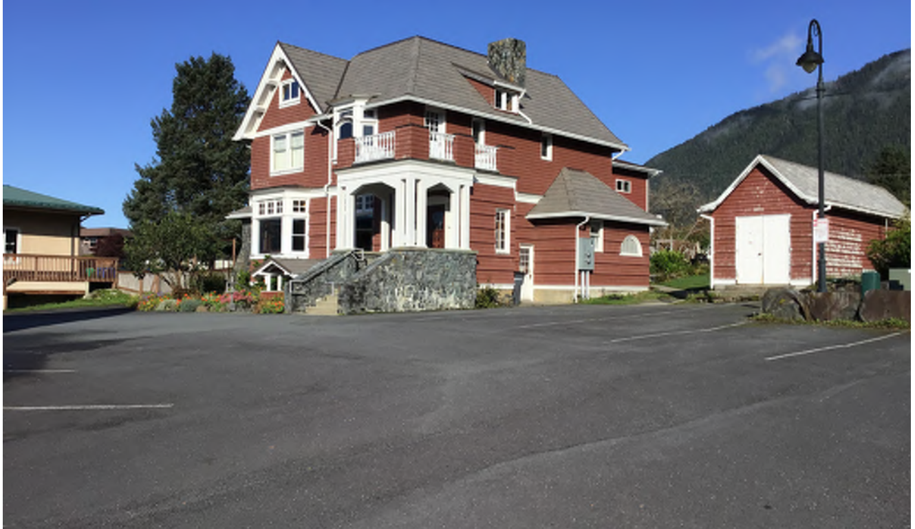
Figure 8.1: The See House is accessed from the asphalt paved driveway with parking that connects to the property entry at Lincoln Street.
