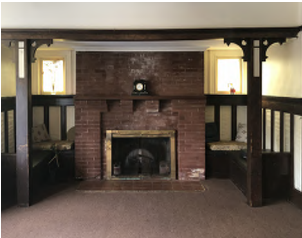
Figure 5.43: Plaster and wainscoting in the inglenook.
