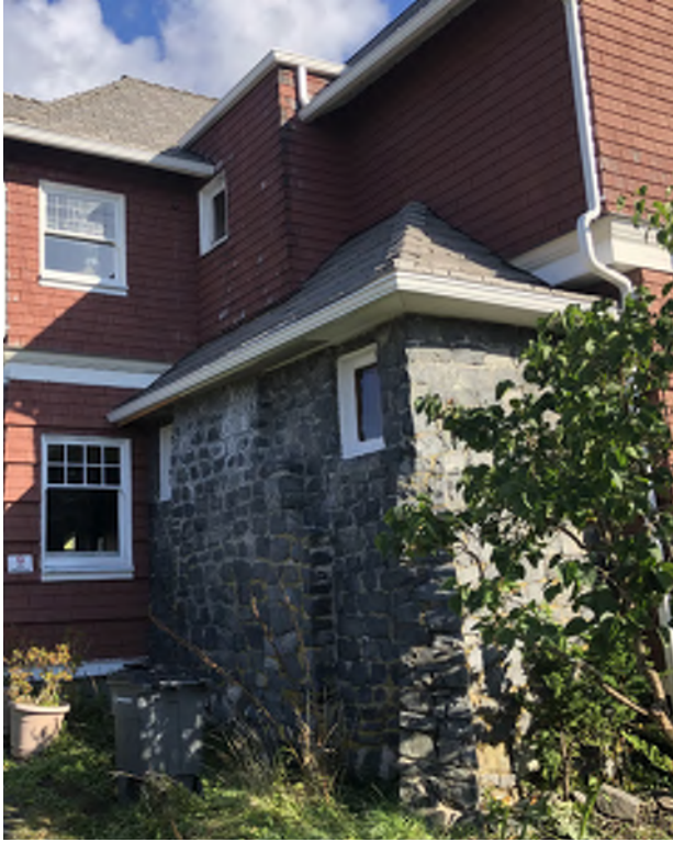
Figure 8.15: Chimney on the west facade above the lower roof was removed.
