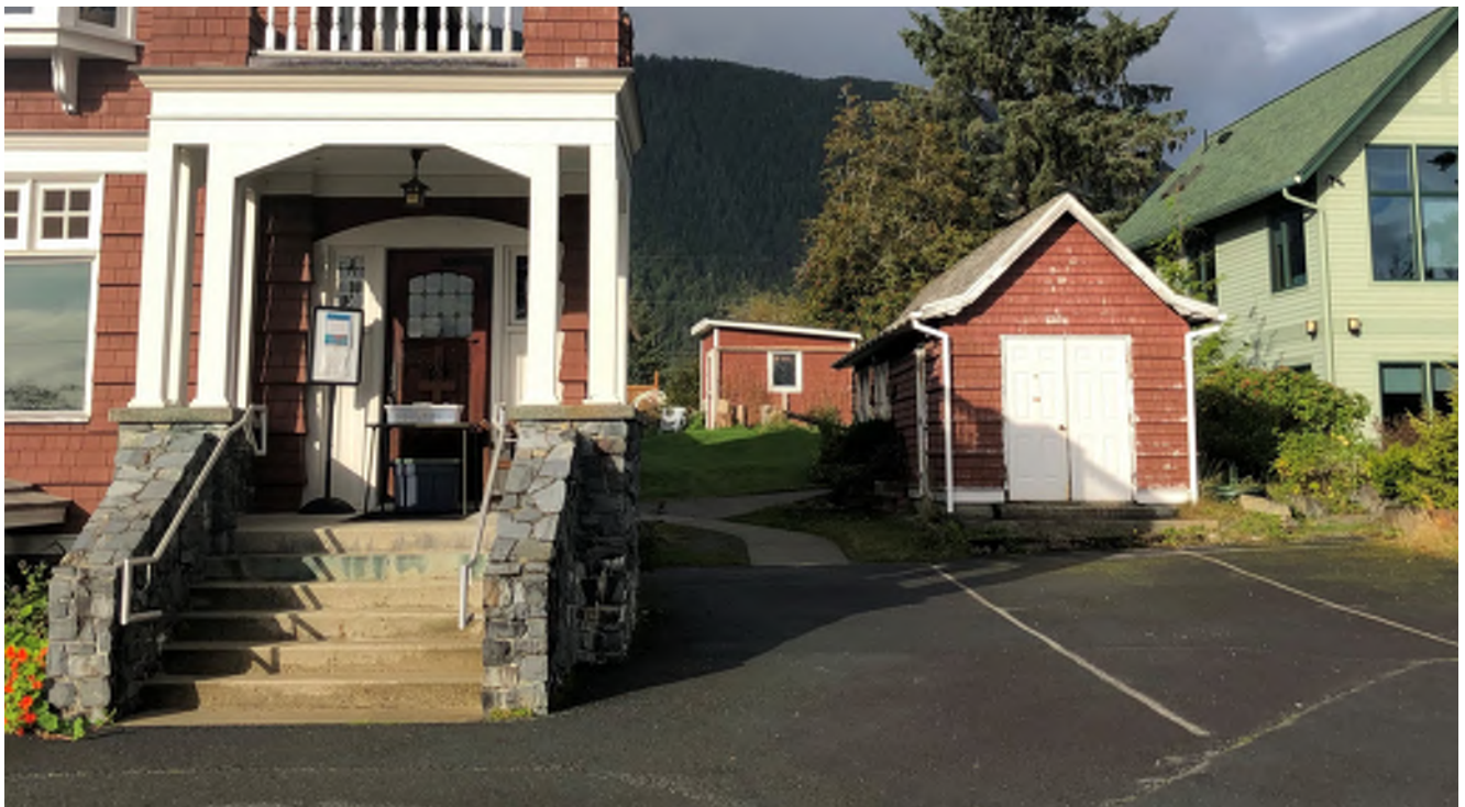
Figure 10.2: Provide a code-compliant accessible parking space including access zone and required signage.
