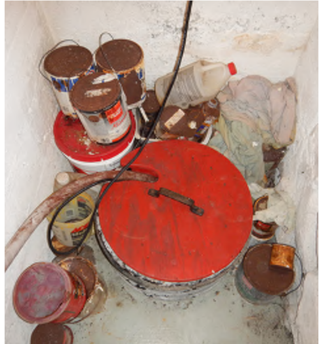
Figure 10.28: Remove hazardous materials stored in basement or install fire lockers for safe containment.
