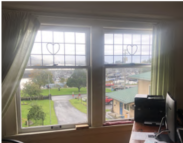
Figure 5.60: The windows in the southwest bedroom (Office).
