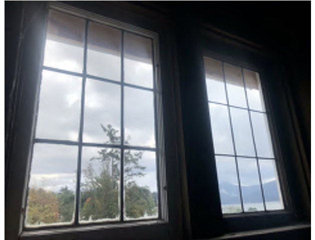
Figure 5.71: The windows at the Attic stair landing.
