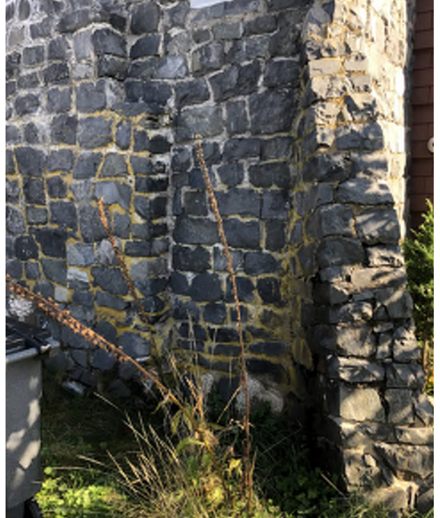
Figure 10.16: Remove biological growth from masonry walls.
