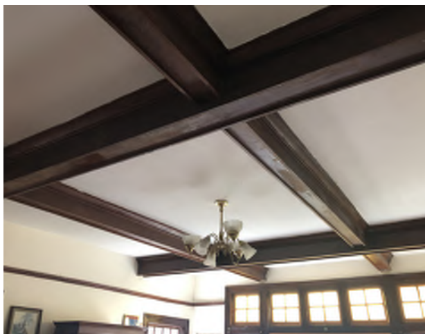
Figure 8.39: Original wood coffered beam and infill panel ceilings in Dining Room.
